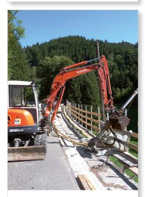
**Verge stabilisation** B33 near Nussbach A capping beam had to be added to an existing retaining wall below a hillside road.
