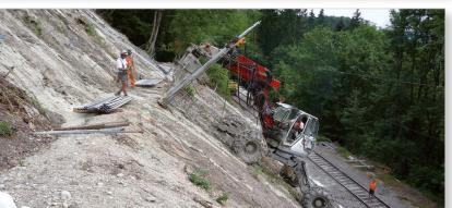
**Slope stabilisation** railway line near Wolfratshausen To protect the tracks against falling rocks, the 25 m high slope was secured with steel wire netting anchored in the ground.
