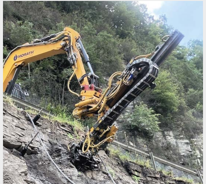
Only small, lightweight plant could be used, and could only work from above
