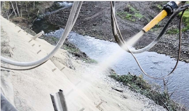
The shotcrete facing is 25 cm thick, up to 50 cm at craters
