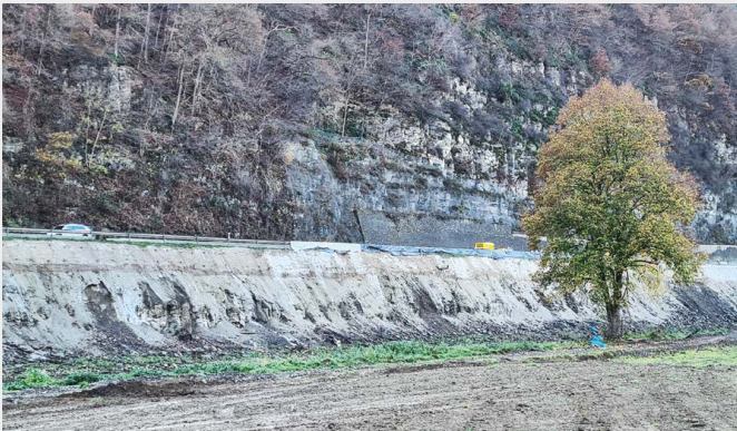
Anchors were installed to secure the slope over a length of about 400 m
