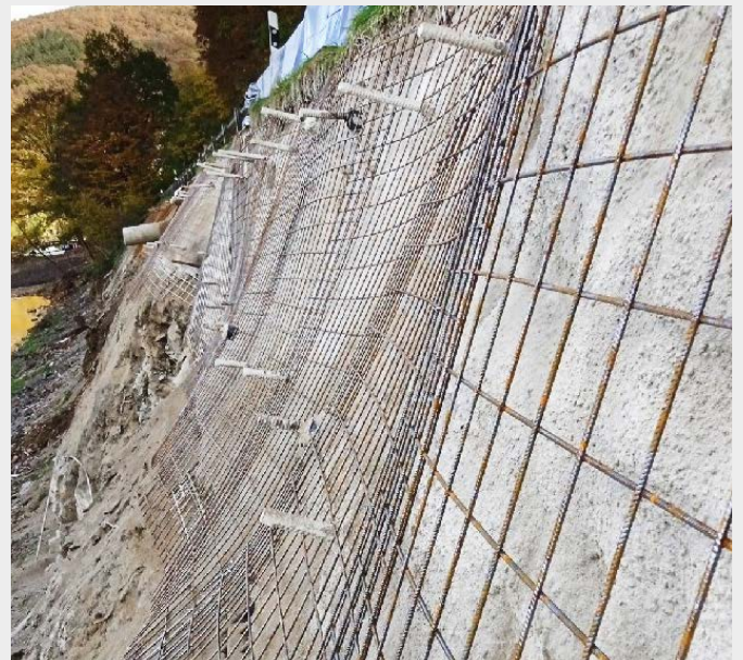
Reinforcement is in the form of two layers of steel mesh
