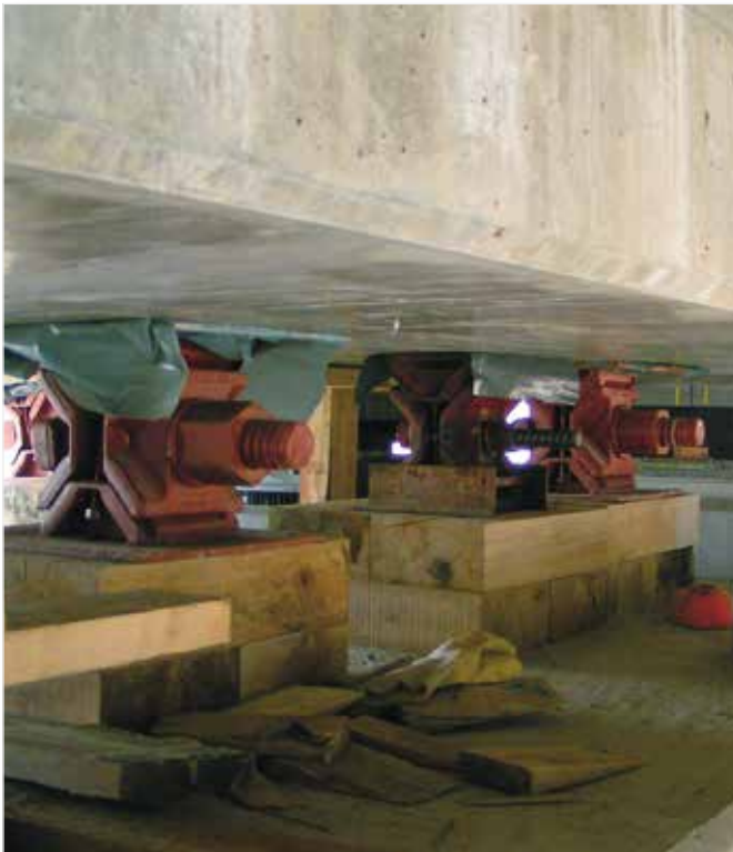
Bridge over River Mulde, Dessau TITAN 500 and TITAN 1000 wedge jacks being used to support precast concrete elements.
